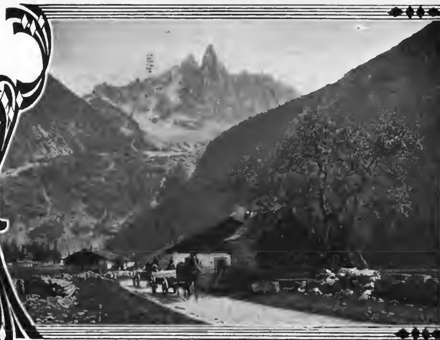
Between Davos and Fillsur, the road built at great expense. The floor of the Valley of Chamounix between Les Praz and Aiguille du Dru
